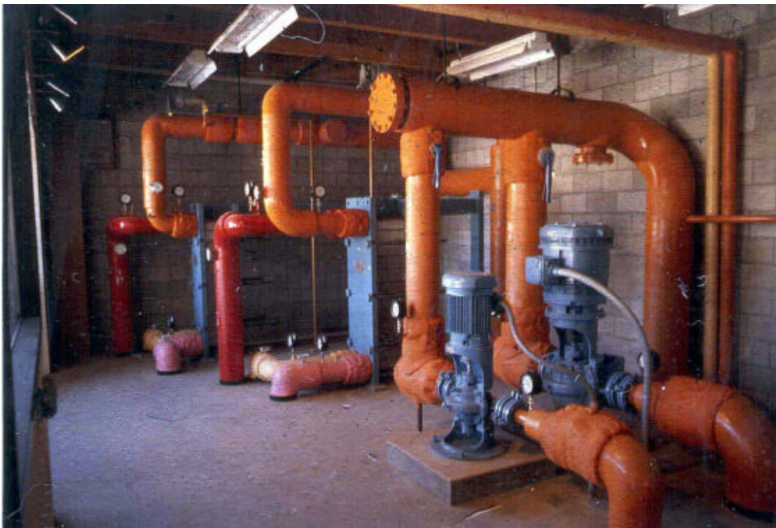
Plate heat exchangers on circulation pumps.
