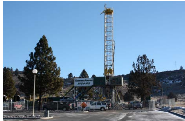
Figure 8: ThermaSource drilling rig on the OIT campus.
