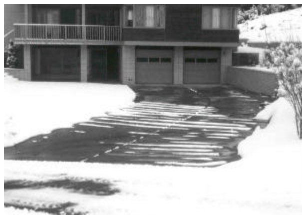
Residential driveways using geothermal water for snow melting. Note that the location of the coils can be determined from the melting pattern.
