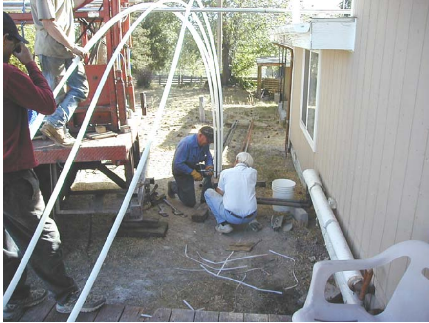
Figure 4. PEX DHE prior to installation, showing the two PEX U-tubes fastened to the black iron pipe of the old DHE, which was used as an installation guide, anchor, and convection promoter.
