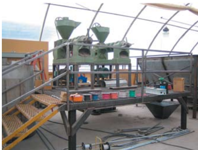
Figure 4. Photograph of equipment for feedstock grinding.
