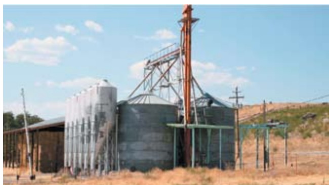
Figure 3. Feedstock grain storage silos.
