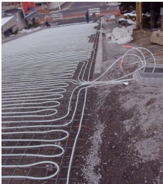
Figure 6. The approach road loops placed latitudinally.
