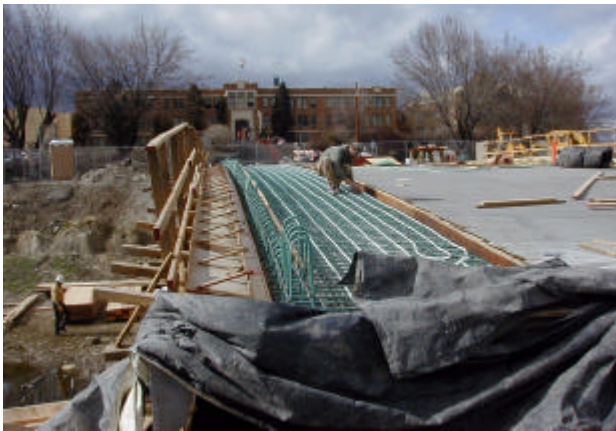
Figure 5. Bridge sidewalk loops.
