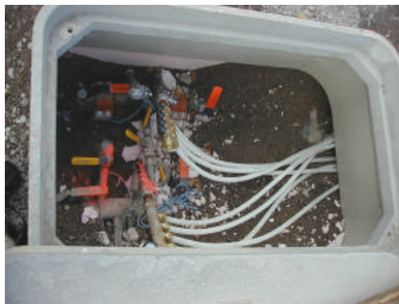
Figure 3. Details of the main control valve box.
