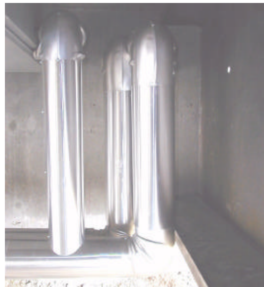
Figure 8. Manifold boxes under the bridge.
