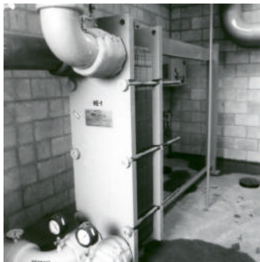
Plate heat exchanger capable of transferring 10 \times 10^6 Btu/r.
