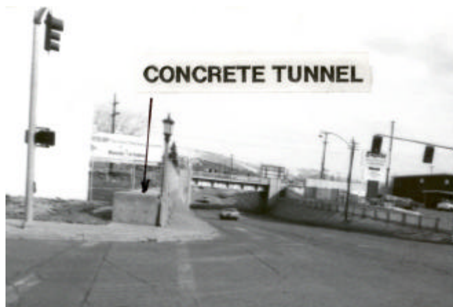
Concrete tunnel above ground for railroad underpass.
