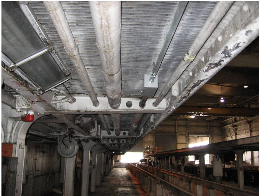
Figure 7. Photograph of old service piping to be retrofitted for overhead radiant heating.
