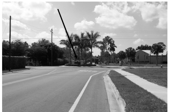
Landscaping enhancement features obstructing sight distance
