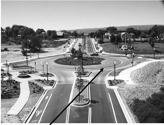
The circulatory roadway should not be wider than 18 feet excluding the truck apron
