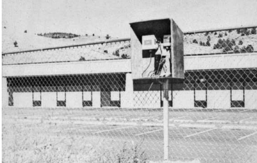
Figure 3. Flow is measured by an electromagnetic flow meter.
