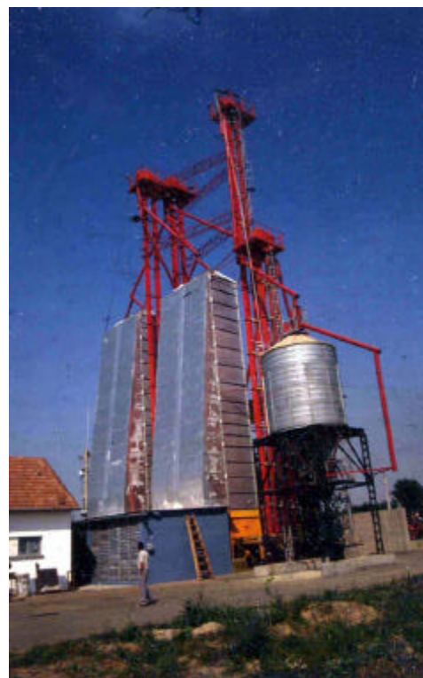
Figure 12. Geothermal grain drier at Szentes.
