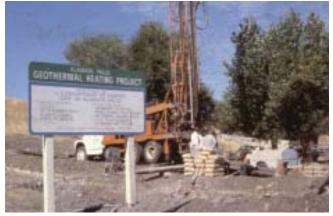
Photo 1: Drilling of CW-1 well (Geo-Heat Center)
