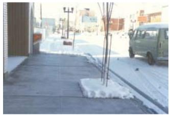
Photo 4: Geothermally Heated Sidewalk Snowmelt (Geo-Heat Center)
