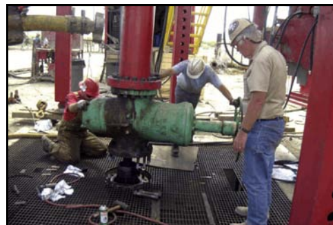
Drill rig workers during the well workover at Raft River, Idaho. (Photo: U.S. Geothermal Inc.)
