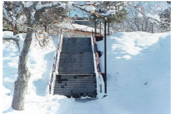
Figure 8. Geothermally snow-melted stairs at the OIT Campus in Klamath Falls, OR.
