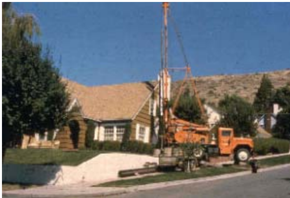
Figure 7. Drilling and installing a downhole heat exchanger at a residence in Klamath Falls.
