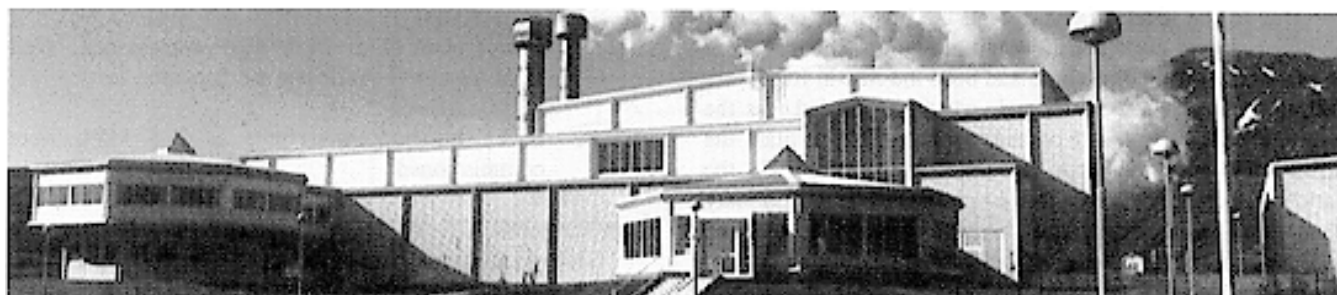
Figure 6. The Nesjavellir power station.
