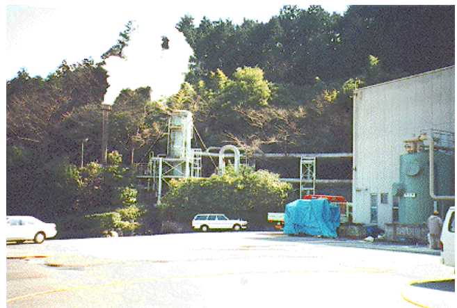
Figure 2. Steam separator.
