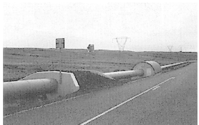
Figure 4. The 800-mm diameter pipeline with a snowmobile crossing.
