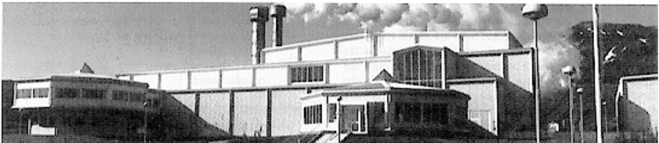
Figure 6. The Nesjavellir power station.
