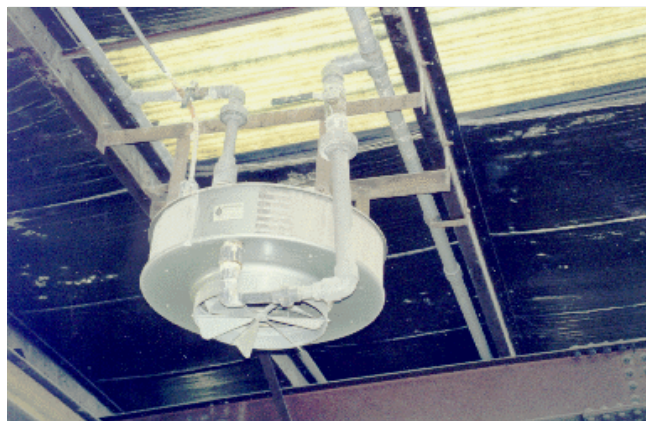
Figure 4. Modine ceiling heater in Philip Motor, Inc.
