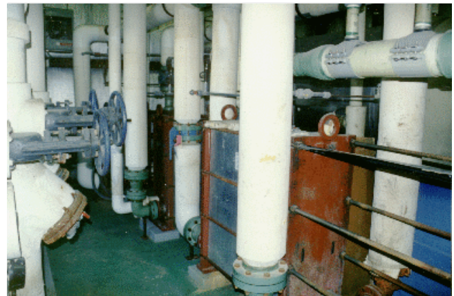
Figure 4. Plate heat exchanger in exchanger building..
