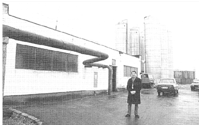
Figure 4. Central heat exchanger building and storage tanks, Oradea district heating system.
