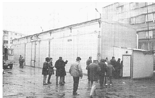
Figure 4. Timber drying facility, Oradea.
