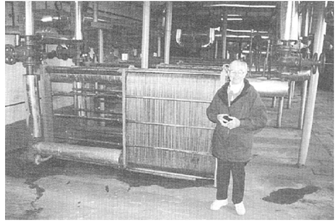
Figure 6. Plate heat exchangers, University of Oradea.
