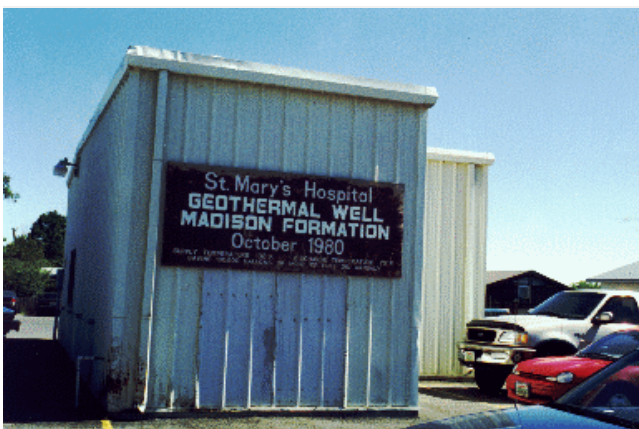
Figure 2. Well house and exchanger building.
