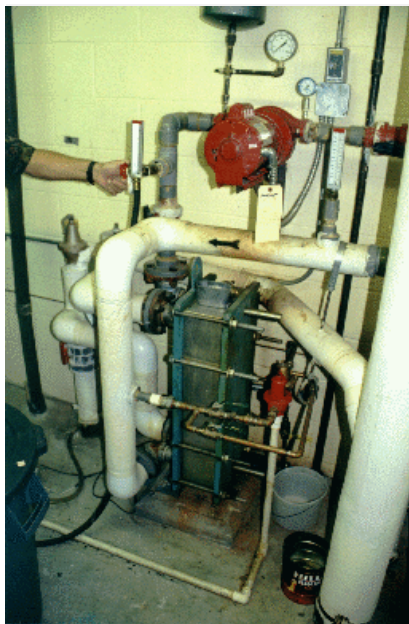
Figure 3. Plate heat exchanger in First National Bank building
