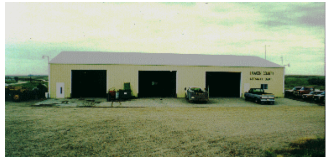
Figure 10. Highway maintenance building.
