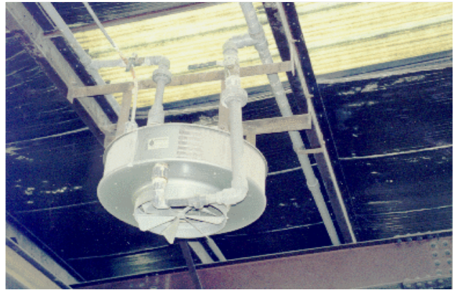
Figure 4. Modine ceiling heater in Philip Motor, Inc.
