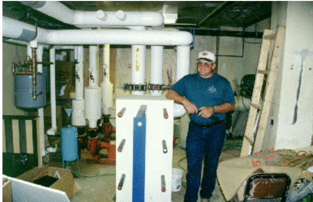
Figure 4. Plate heat exchanger in basement of Discovery Center.
