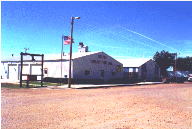
Figure 10. Fire station, Tim-Buck-2 Bar and Restaurant.
