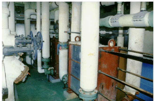
Figure 4. Plate heat exchanger in exchanger building..
