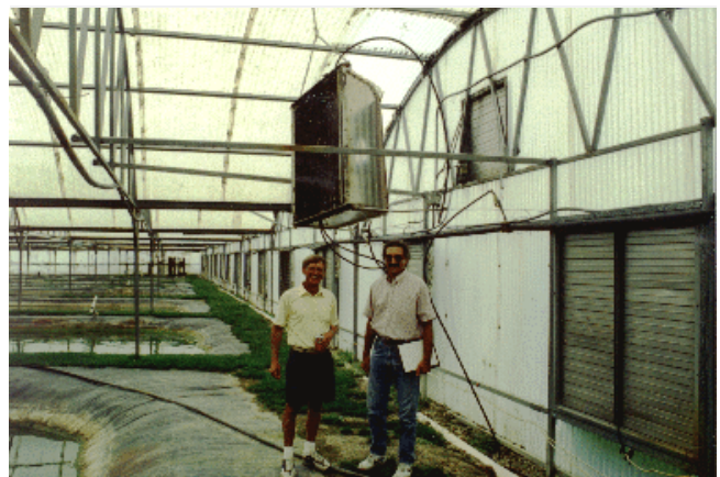
Figure 15. Unit heaters with Pat Seager, manager and Steve Wegman.
