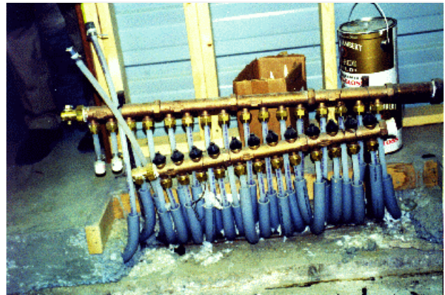
Figure 5. Floor heating loops in the Philip Fire Department.
