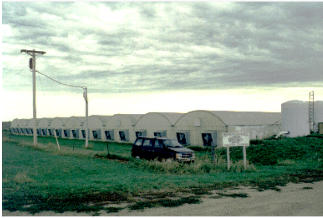
Figure 11. Greenhouses with storage tanks on right.
