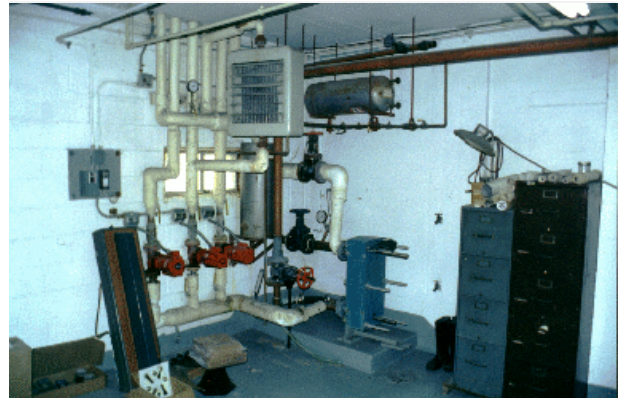
Figure 9. Plate heat exchanger and unit heater in water treatment building.
