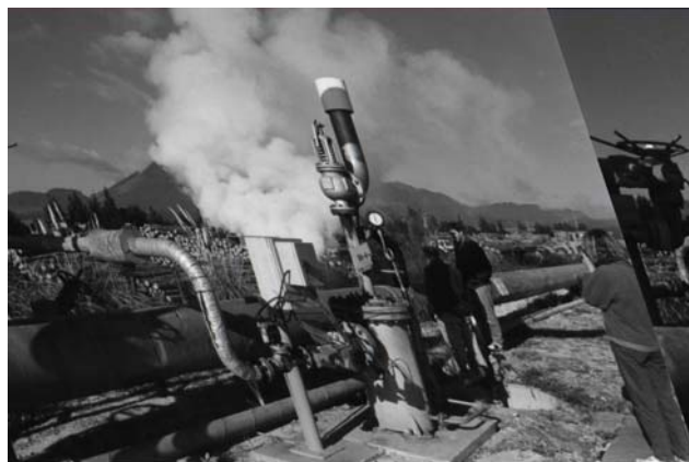
Figure 3. Separator on two-phase line with pressure control valve.
