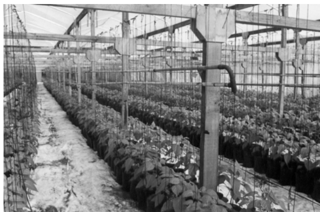
Figure 1. Older greenhouse with Capsicum (green peppers) plants and heating pipes (bottom one is condensate return)
