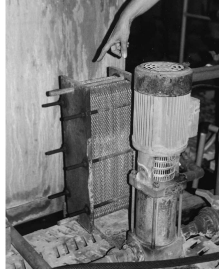
Figure 2. Plate heat exchanger inside the facility.
