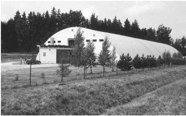
Figure 4. Overview of the building..
