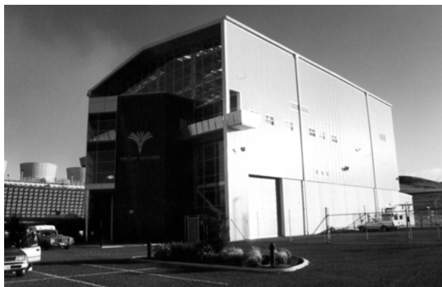
Figure 5. Mercury Geotherm turbine-generator building.
