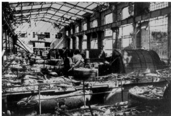
Figure 1. Destroyed Lardarello No 2 Station Turbine Hall.
