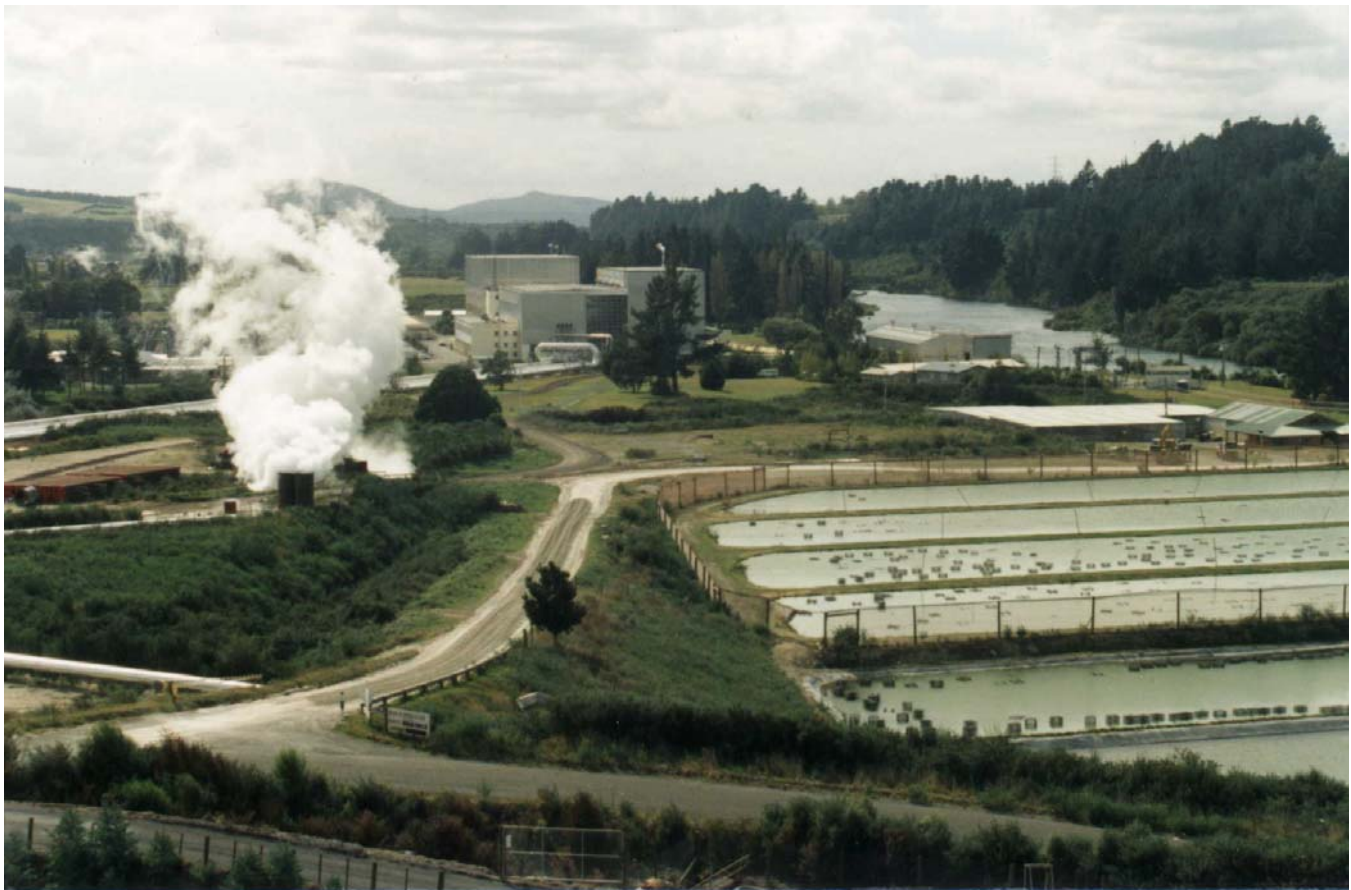
Figure 1. Prawn Park with Wairakei Power plant and Waikato River.
