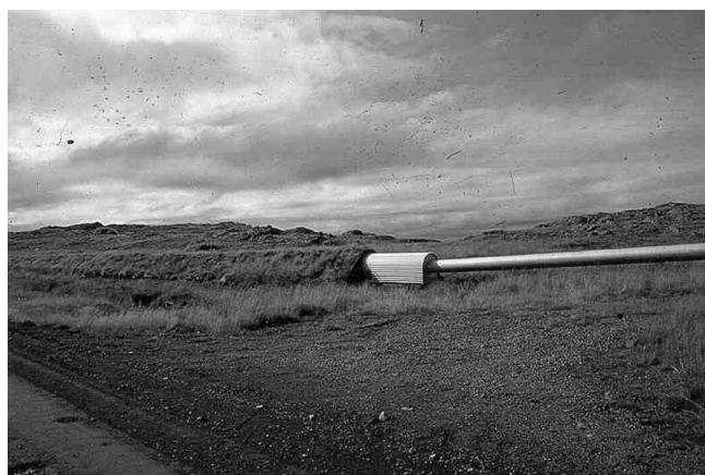
Figure 4. Aboveground steel insulated pipe and buried asbestos cement pipe.
