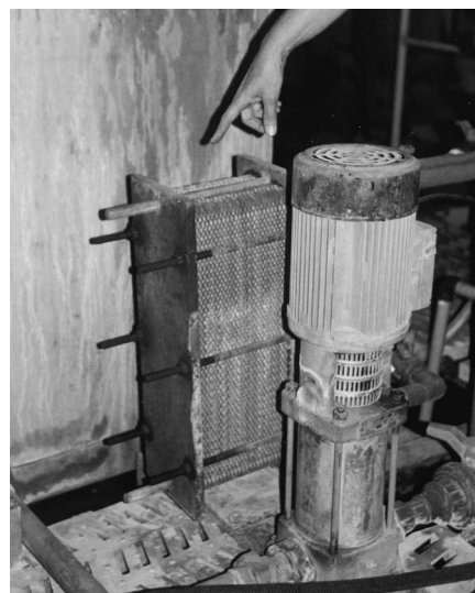
Figure 2. Plate heat exchanger inside the facility.
