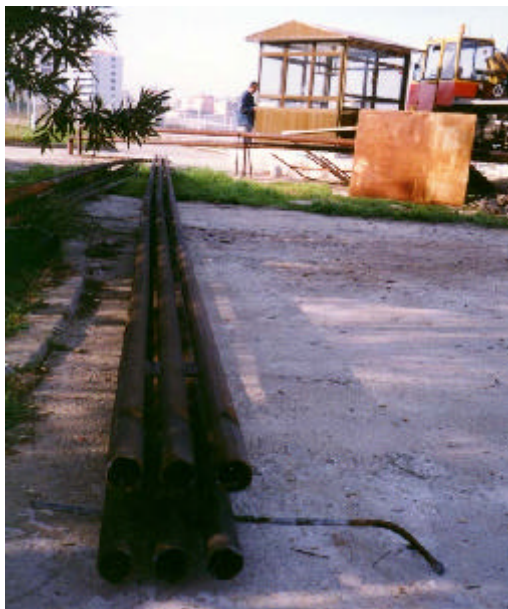
Figure 3. Downhole heat exchanger pipes used for one well at Balçova.
