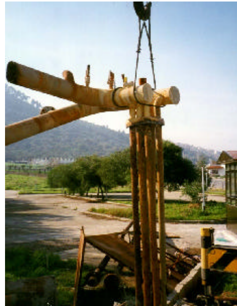
Figure 2. Details of header pipe attached to the top of the DHE in Balçova.
