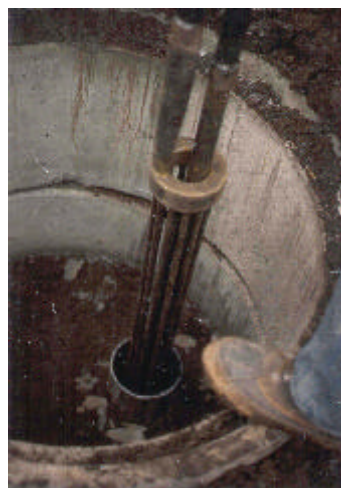
Figure 5. Test project using multiple loops being lowered in the well.
