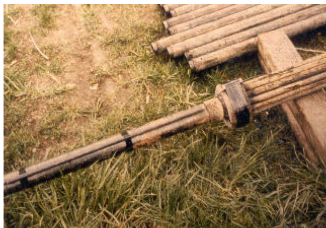
Figure 4. Details of the multiple loop installation with circular header.
