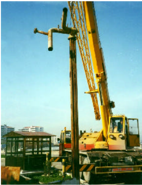
Figure 1. Downhole heat exchanger being removed from a well at Balçova.
