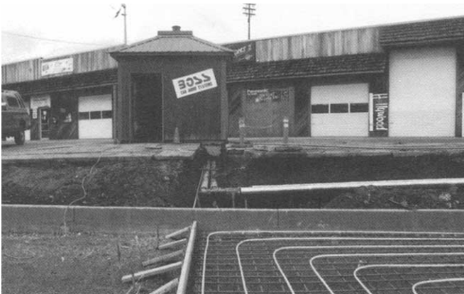
Figure 9. End of project and pump house in background.
