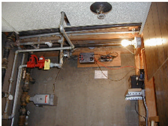
Figure 5. Motorized control valve, solid state controller and expansion tank - the pressure reducing and pressure relief valves in the foreground.
