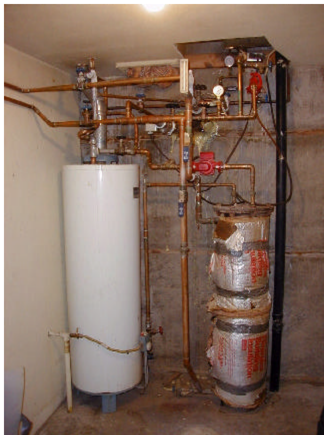
Figure 8. The interior mechanical system showing the domestic hot water shell-and-tube heat exchanger on the right and the water storage tank on the left. The pipes from the DHE enter at the top-center of the photograph. Circulation pumps can also be seen in the center top.
