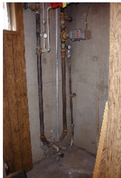
Figure 4. Two loops from the DHE entering the home from the well—one for space heating and the other for domestic hot water.
