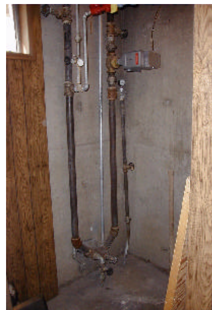
Figure 4. Two loops from the DHE entering the home—one for space heating and the other for domestic hot water.
