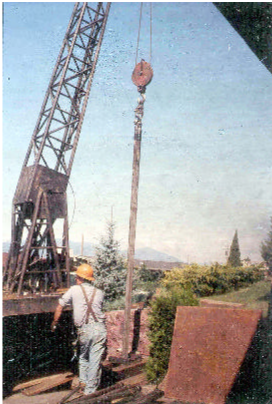
Figure 2. Placing a 2-in. (5-cm) diameter loop in a well.
