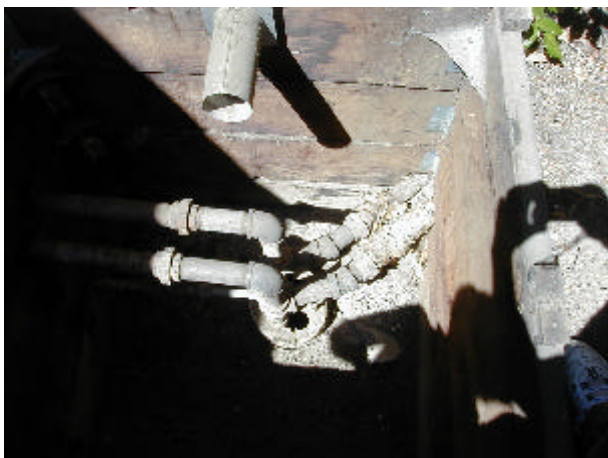
Figure 2. Well with three DHEs, a single 2-inch (5-cm) pipe used for space heating and two 3/4-inch (2-cm) pipes used for domestic hot water.
