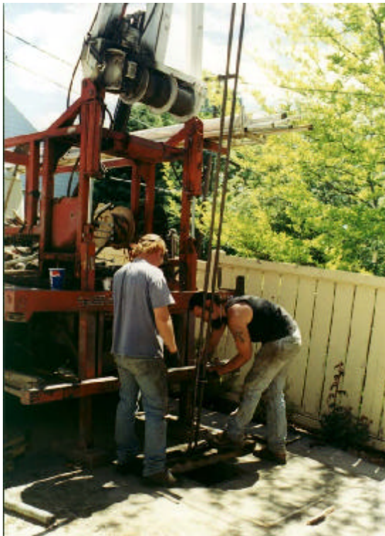
Figure 5. Installing the 3/4-in. (2-cm) diameter domestic hot water heating loop.
