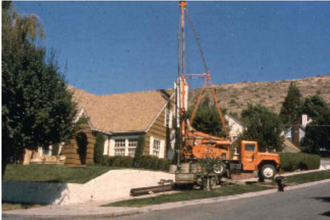
Figure 1. Drilling a residential geothermal well with a cable drilling rig.
