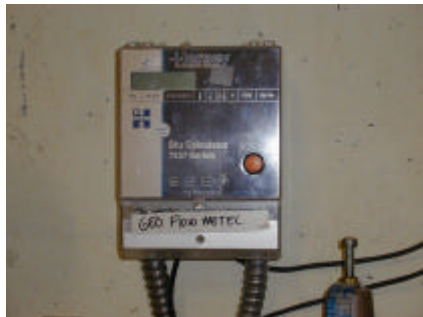
Energy and flow totalizer in Courthouse.
