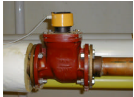
Turbine flow meter in Courthouse.
