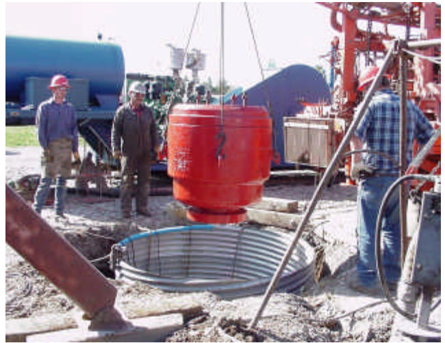
Figure 2. Blowout preventor being installed.
