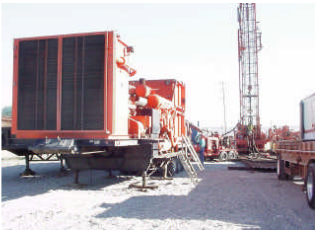
Figure 5. Compressor for blowing out the well.
