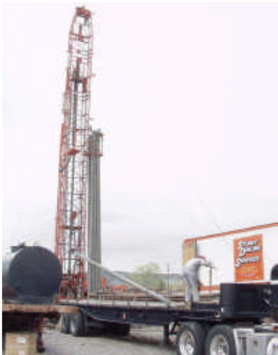
Figure 1. Drilling rig setup.
