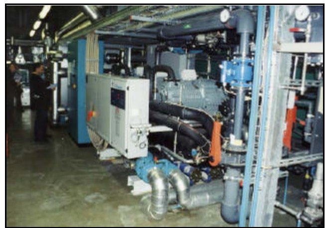
Figure 6. Heat pump equipment room.
