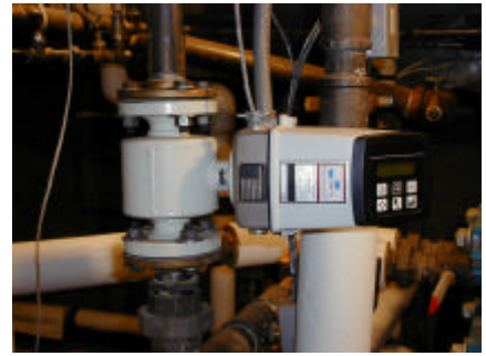
Magnetic flow meter in Library.
