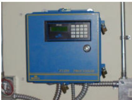
Energy and flow totalizer in Government Center.
