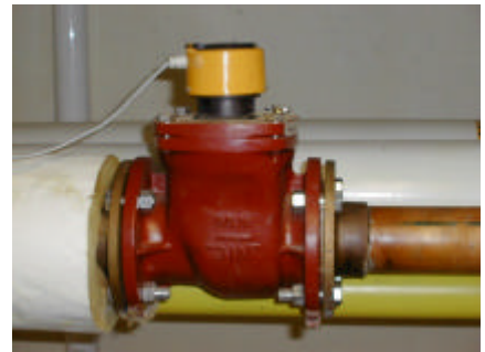
Turbine flow meter in Courthouse.
