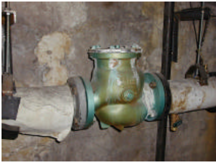
Original turbine meter (no longer functional).
