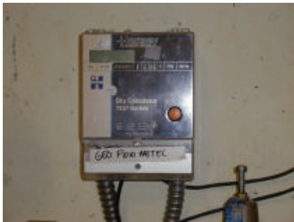
Energy and flow totalizer in Courthouse.
