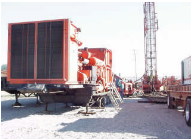
Figure 5. Compressor for blowing out the well.
