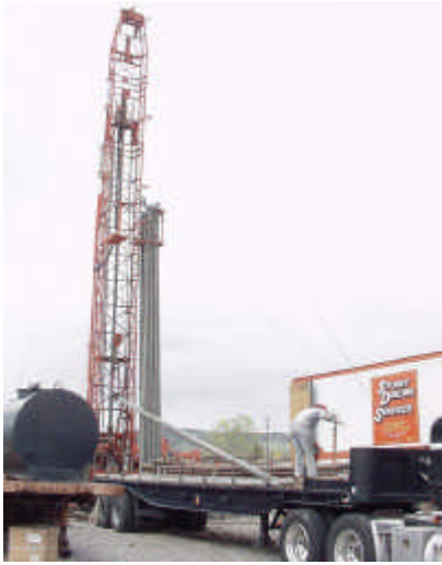
Figure 1. Drilling rig setup.
