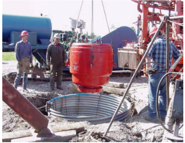
Figure 2. Blowout preventor being installed.
