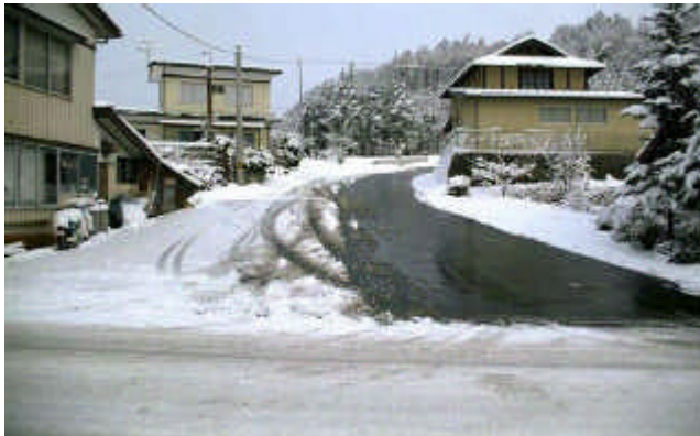
Figure 4. Snow-melting condition at the lower section of the road on February 13, 1996.
