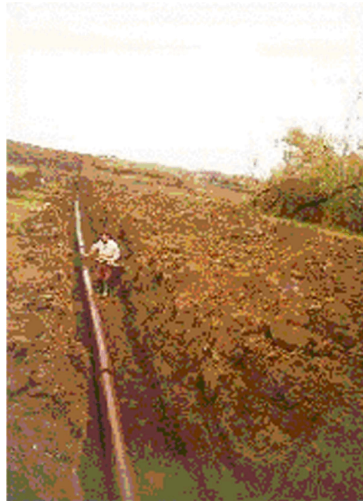
Figure 3. Pre-insulated FRP pipes for geothermal water transportation.
