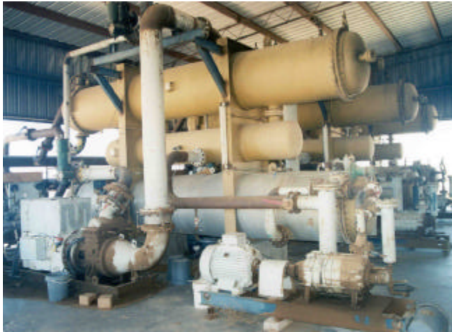
Photo 3. ORMAT/SPS binary power units.
