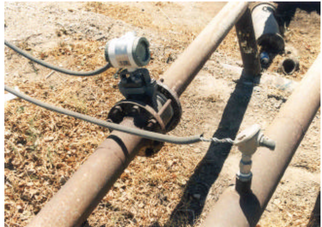
Photo 5. Energy meters at Burgett's Greenhouses.
