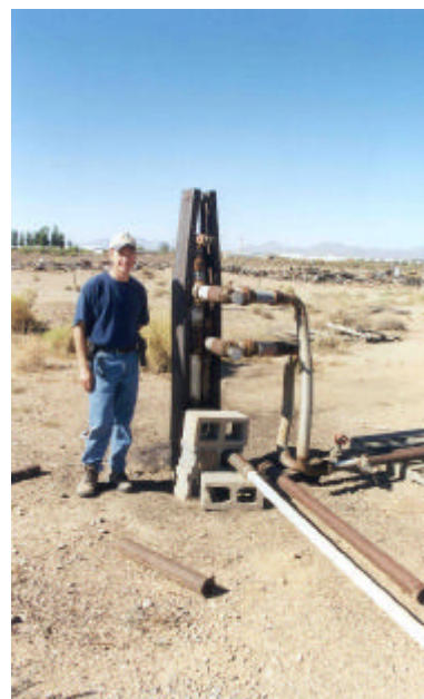
Photo 9. Downhole heat exchanger system with Manager/Owner Damon Seawright.
