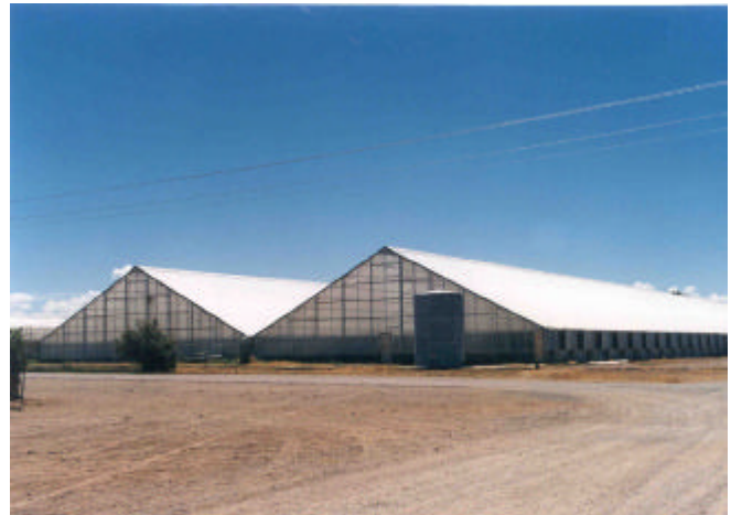
Photo 1. 80-ft by 400-ft Lord and Burnham greenhouses.
