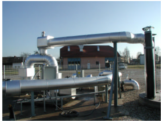
Figure 4. Well 1A with pump house.
