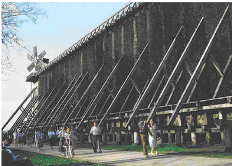
Figure 6. Ciechocinek Spa – wooden cooling tower for spraying brines and creating an ocean-like microclimate (Source: Internet page www.ciechocinek.pl ).
