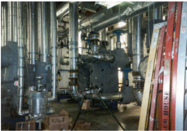
Figure 5. Space heat exchanger, located in prison boiler room (photo: Mark A. Miller).
