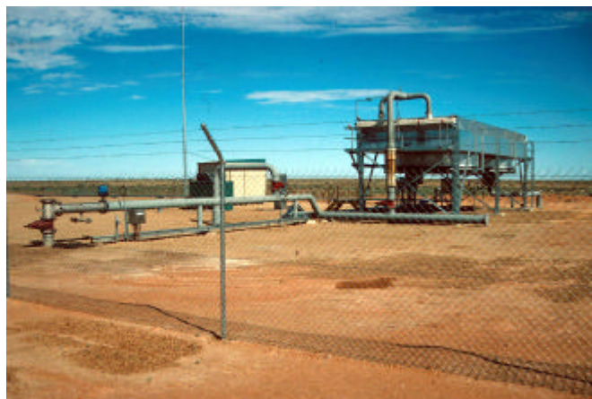
Figure 2. Cooling tower in the Borefield B of the Olympic Dam Mine, SA.
