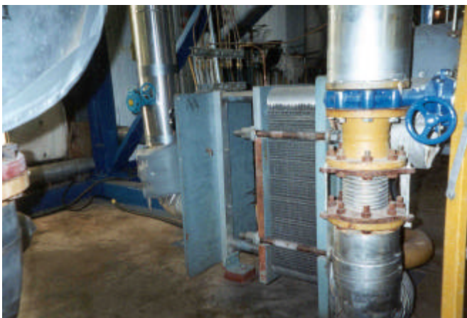
Figure 6. Domestic heat exchanger (photo: Mark A. Miller).
