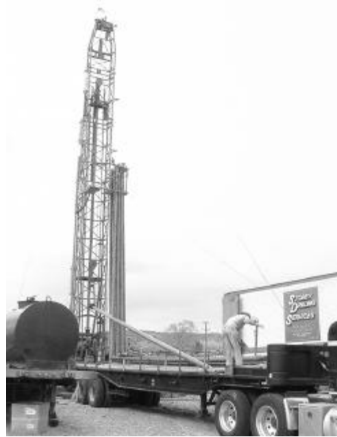
Figure 3. Drilling the well.
