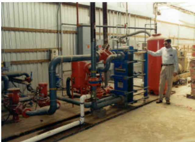
Photo 4. The existing plate heat exchanger (Jim Witcher).
