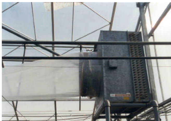
Photo 4. Modine heater with poly tube.
