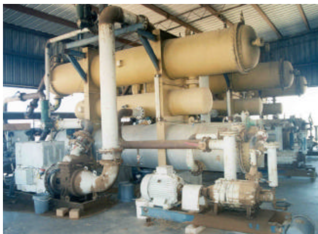
Photo 3. ORMAT/SPS binary power units.
