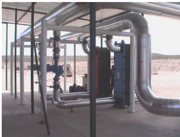
Photo 3. The two new plate heat exchangers.
