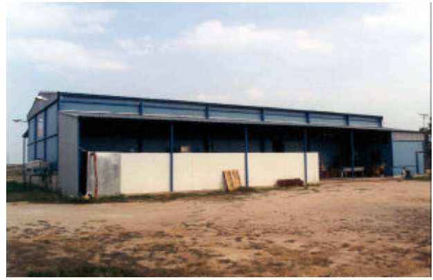
Figure 2. Overview of building and drier (the long, light colored box)
