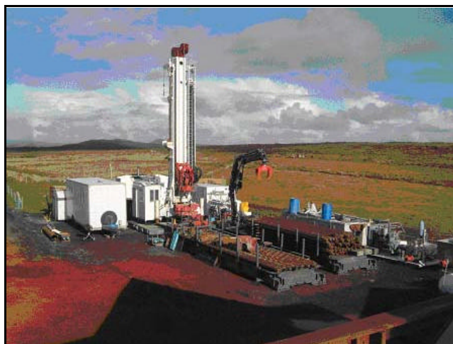
Figure 5. Dilling rig "Saga" at location in Grímsnes.
