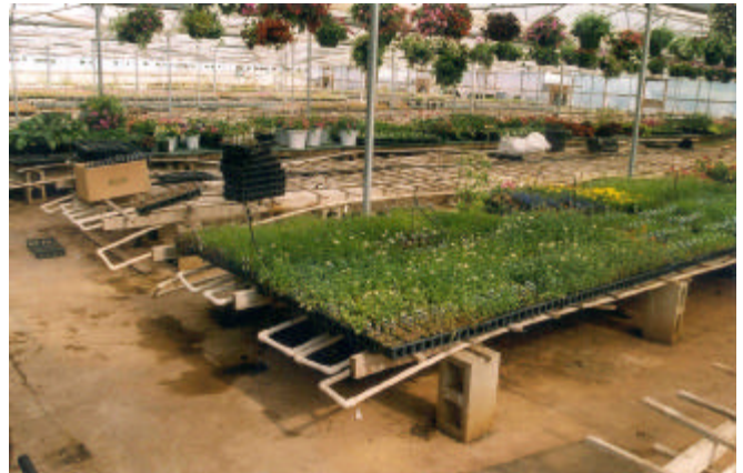
Interior of a greenhouse with the PVC heating pipes under the benches.
