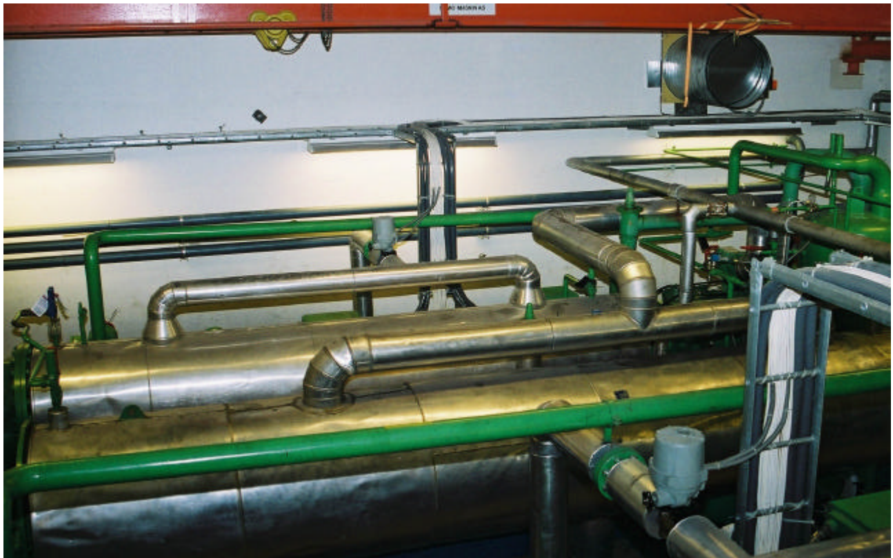
The Bodø system’s heat pump consists of two separate aggregates with shell-and-tube condensers and evaporators.
