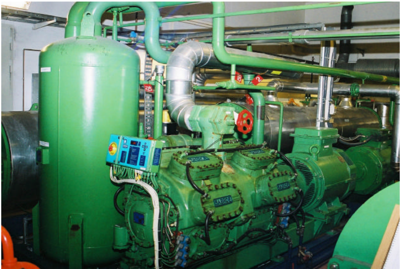
In the Bodø district heating system, vapor enters this low-pressure compressor and then the barrel-like “inter-stage receiver,” where temperature is reduced before the vapor continues into the high-pressure compressor.
