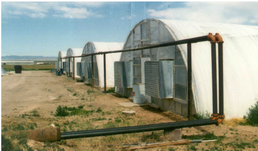
Castlevalley greenhouses showing geothermal water supply lines.
