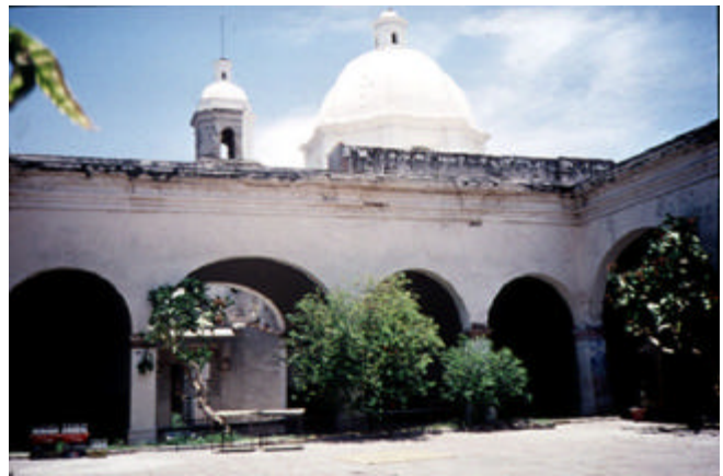
Photo 5. Interior patio with church dome in background.
