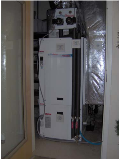
Figure 3. Photograph of a 6-ton, water-air, vertical heat pump and flow center.
