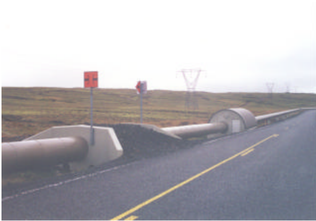
Figure 5. The 800-mm diameter pipeline with a snowmobile crossing.
