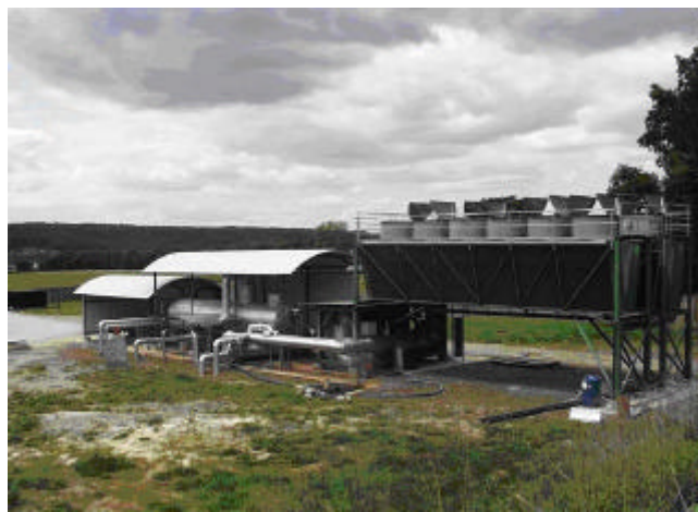
Figure 4. ORC installation at well Blumau 2.
